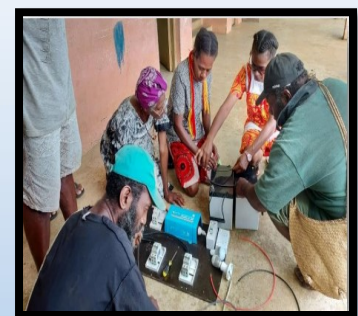
Figure 2: Participants from Melsisi in Pentecost (Vanuatu) conducting wiring exercise on the solar home system demonstration kit.
